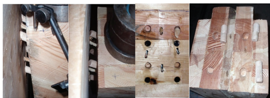
Fig. 11: Failed connection with a detail of partially pulled up wood screws and pushed oak dowels \varnothing 16 mm to the stringer and the front board.
